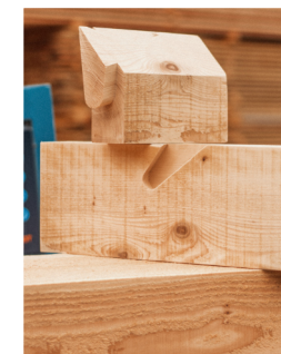
Angled dovetail joint
