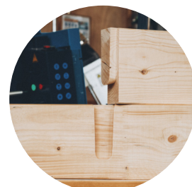
Male and female dovetail joint
