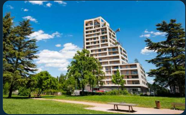
Plein Ciel • Strasbourg (67) Denu & Paradon Architecture
