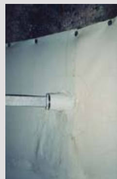
19 – Watertight seal around a steel insert crossing the geomembrane (Mont Jovet tunnel, Italy).
