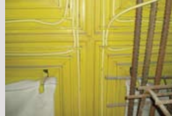
11 – Post-grouting arrangement at a waterstop cross joint (Dobrovskeho tunnel, Czech Republic).
