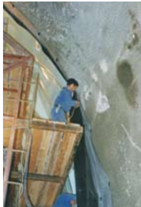
7 – The geomembrane being placed onto the geotextile already secured to the sprayed concrete substrate (Lisbon metro tunnel, Portugal).
