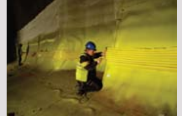
12 – Longitudinal compartment seal made by welding the waterstop to the geomembrane. The waterstop is then embedded into the concrete inner lining (Klimkovice tunnel, Czech Republic).
