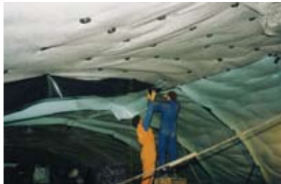
8 – In the foreground the geotextile fixed to the substrate. In the background the geomembrane heat welded to the roundels (Lisbon metro tunnel, Portugal).
