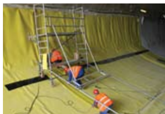
10 – Installation of the circumferential waterstop onto the geomembrane in the tunnel invert (Dobrovskeho tunnel, Czech Republic).
