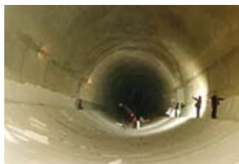
9 – Installation of the geomembrane in the invert (Capo Calava' tunnel, Messina-Palermo highway, Italy).
