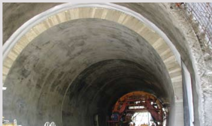
20 – Inner lining on the Krasikov tunnel, Czech Republic.
