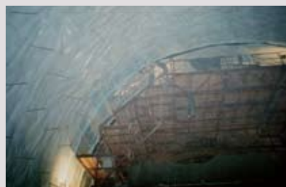
18 – Anchoring steel bars protruding through the geomembrane (Baixa Chiado, Lisbon metro tunnel, Portugal).
