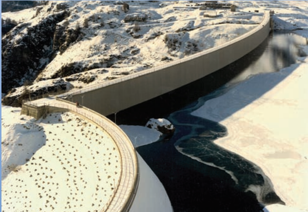
Cignana dam rehabilitated with CARPI SYSTEM (1988). The geomembrane system in 2011 is in full service.
