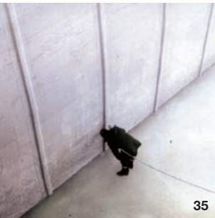
35 - SIBELON® CNT geocomposite can resist impact of thick ice covers. Ice does not stick to the geomembrane, which is therefore not affected by shear forces.
