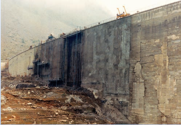
The upstream face of Cignana dam, deteriorated by freezing and thawing cycles, before rehabilitation.
