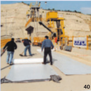
39 - The sacrifice layers span the area over the fissure that is within the perimeter seal.
