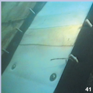
44 - The perimeter seal is made by puncturing the waterproofing PVC geocomposite over the anchor rods and by compressing it on the RCC with stainless steel batten strips and rubber gaskets.
