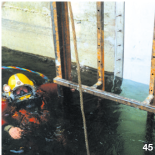
45 - The drilling template facilitated the final underwater work of installing the stainless steel batten strips and of tightening the nuts to achieve the seal at the perimeter. The photo details the holes in the steel frame corresponding to the tightened nuts at the perimeter of the dry part.
