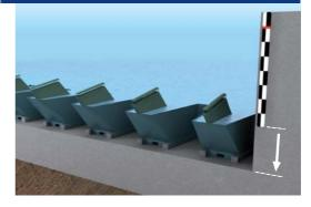
Installing Fusegates on lowered spillway sill maintains initial storage capacity while ensuring the discharge of the revised design flood.
