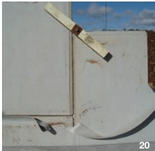
20/21 - Welding of PVC geomembrane strips waterproofing the perimeter of the precast concrete panels.
