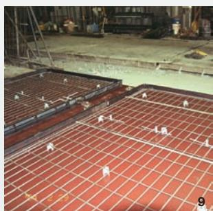
9 - Placement of reinforcement and insert plates before casting conventional concrete in the formwork.
