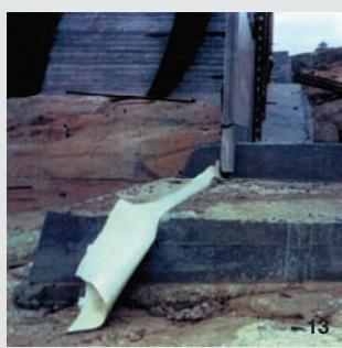
13 - The geomembrane key prior to connection to the starter panel.
