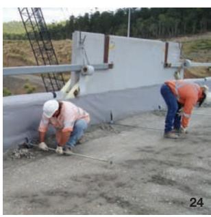
24 - Burnett River dam (35 m), 2005 Australia: the anchoring rods being installed on the panels.
