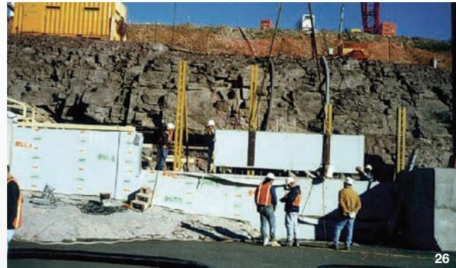
26 - Hughes River dam (30 m), 2001 USA: placement of precast panels.
