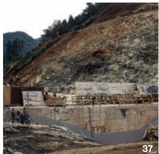
37/38 - Waterproofing of the perimeter plinth: installation of the geocomposite, and concreting. Use of waterstops avoided.
