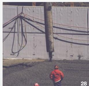
28 - Hughes River dam (30 m), 2001 USA: placing of RCC against panels.
