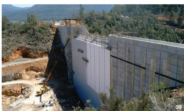
39 - Meander dam, designed with low cementitious content concrete RCC mix and a waterproofing geomembrane to save the cost of high cementitious content mix.
