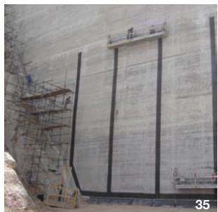
35 - Vertical strips of geonet being installed at Taishir RCC dam, 2007 Mongolia (option with external profiles).
