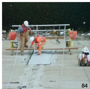
83 - Strawberry CFRD (43 m), 2002 USA: the failing joints between face slabs.
