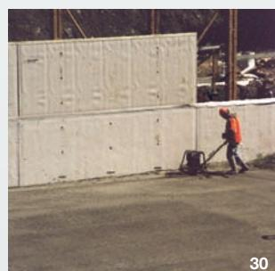
30 - Adjacent to the geomembrane, the RCC is compacted with vibrating plate compactors to avoid damaging the synthetic liner.
