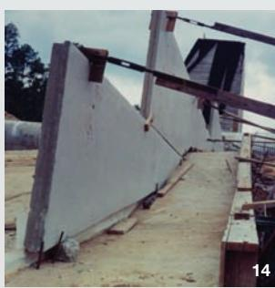
14 - The geomembrane key welded to the starter panels.
