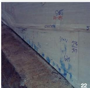
22/23 - Watertightness of all welds is inspected prior to RCC placement.
