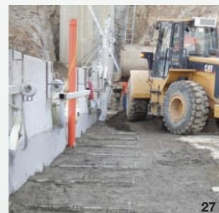
27 - The anchoring rods being embedded in the RCC lifts.
