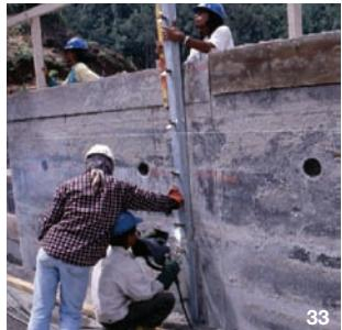
33 - The vertical anchoring steel profile that works as a free-flow drainage conduit is placed against formwork (option with embedded profiles).
