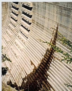
92 - The crack dried out a few hours after installation of CARPI external waterstop (wet on the left and dry on the right).
