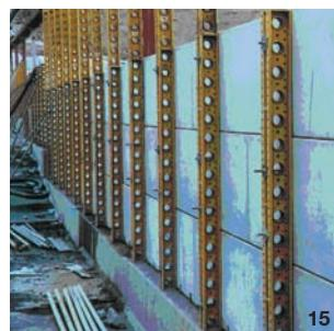
15 - Supports for stabilization of the panels during RCC placement.
