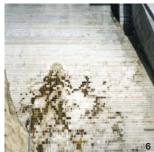
1/2 - Formation of cracks on the upstream face of RCC dams, creating a new unprotected joint in the dam.
