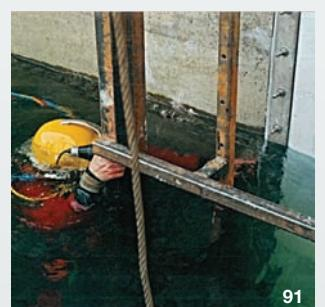
90 - The waterproofing system was installed on a total length of ~ 20 m in the dry from crest level at 227.50 m to elevation 225 m, and underwater from elevation 225 m down to elevation 208 m.
