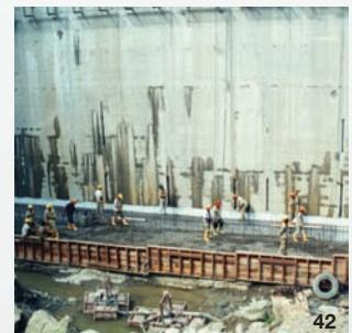
41 - Miel I dam (188 m), 2002 Colombia: completing waterproofing and casting of perimeter plinth at bottom.
