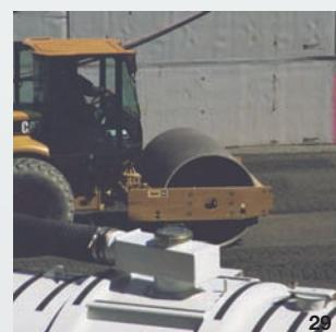
29 - Careful compacting of RCC close to the geomembrane.
