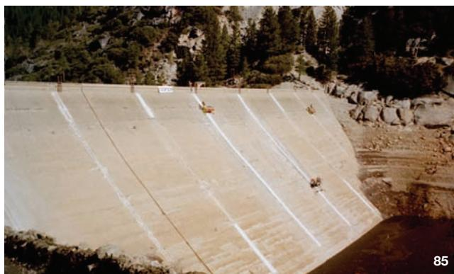
85 - Joints between face slabs of the CFRD were waterproofed with CARPI external waterstop system.
