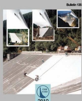
Miel I RCC dam, 2002 Columbia, pictured on the cover of the ICOLD Bulletin 135 (2010) Geomembrane Sealing Systems for Dams..
