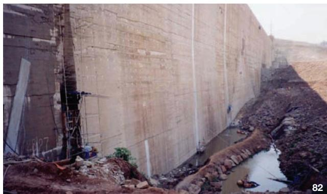
82 - CARPI patented external waterstop was installed on the new joints and on the cracks.
