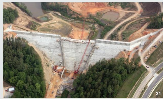
31 - Hickory Log dam (55 m), 2007 USA. Highest RCC dam in the world with Winchester system.
