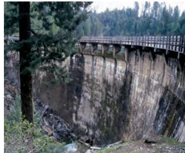
◀ Watertight perimeter seals avoid water infiltration behind the geocomposite. At Olai Dam, Italy , Carpi's external waterstops installed on three failing joints reduced total leakage from > 65 l/s to 0.33 l/s.
