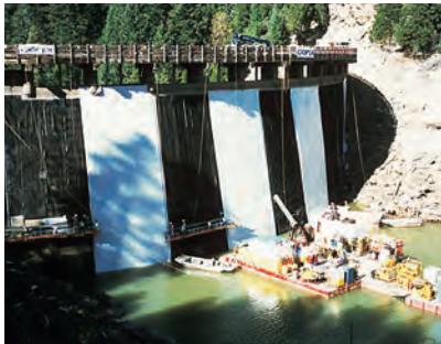
▲ Turimiquire CFRD, Venezuela (113 m high): A Carpi geocomposite system was installed to a depth of 65 m. Construction was staged to first repair the areas causing most leakage. Dramatic reduction of leakage was achieved after underwater installation of the geocomposite system on about 1/5 of the upstream face.
