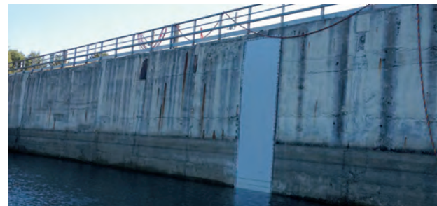
◀ Watertight perimeter seals avoid water infiltration behind the geocomposite. At Olai Dam, Italy , Carpi's external waterstops installed on three failing joints reduced total leakage from > 65 l/s to 0.33 l/s.
