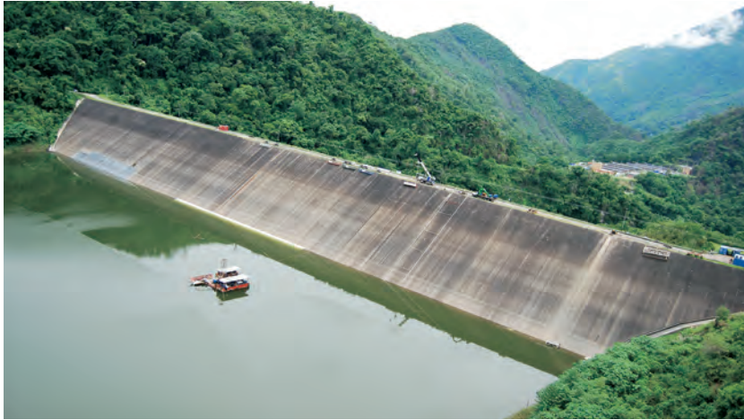
▲ Turimiquire CFRD, Venezuela (113 m high): A Carpi geocomposite system was installed to a depth of 65 m. Construction was staged to first repair the areas causing most leakage. Dramatic reduction of leakage was achieved after underwater installation of the geocomposite system on about 1/5 of the upstream face.
