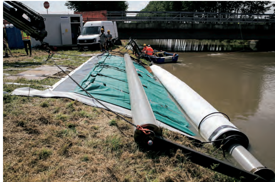
▲ The rolled mattress can be deployed using a customised hydraulic trolley.
