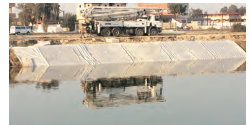
▲ Once the Sibelonmat® is in place underwater, workers fill each section with grout. The tensile properties of the lower geomembrane and the heavy weight of the grout keep the preparation of the subgrade to a minimum.
