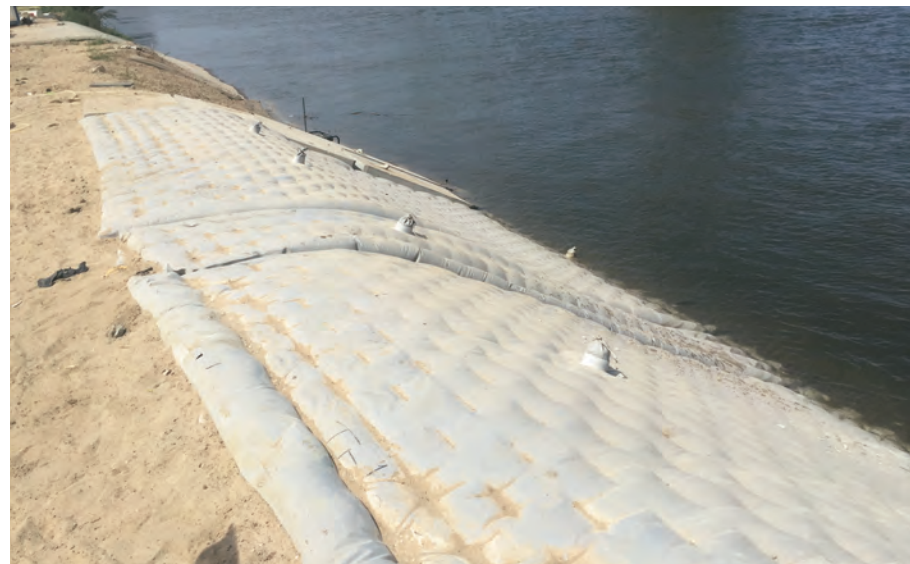
▲ Once completed, a Sibelonmat® provides a strong barrier to water seepage. No interruptions to dam/canal operations are required for its installation.
