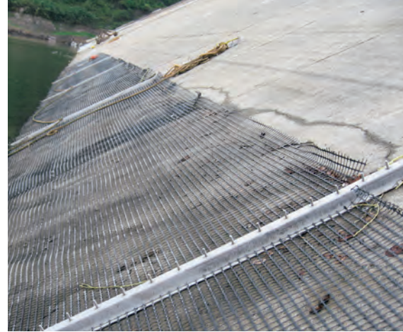
▲ Geogrids and geotextiles are used for support over large cavities and to provide anti-puncture protection. This keeps surface preparation to a minimum. Here, a geogrid is installed at the waterline.
