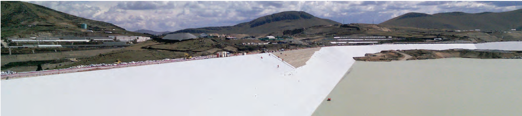
▲ Carpi completing installation of geocomposite on a new tailings dam.
