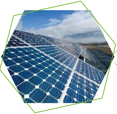
Large solar power plant
