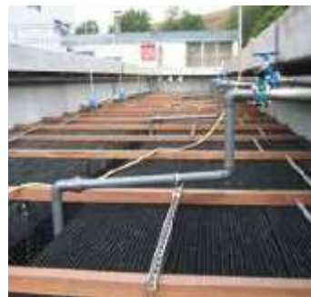
installation de BIOdek® IFAS
