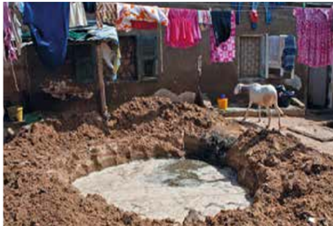
Valve water from a septic tank overflowing in the rising zone
