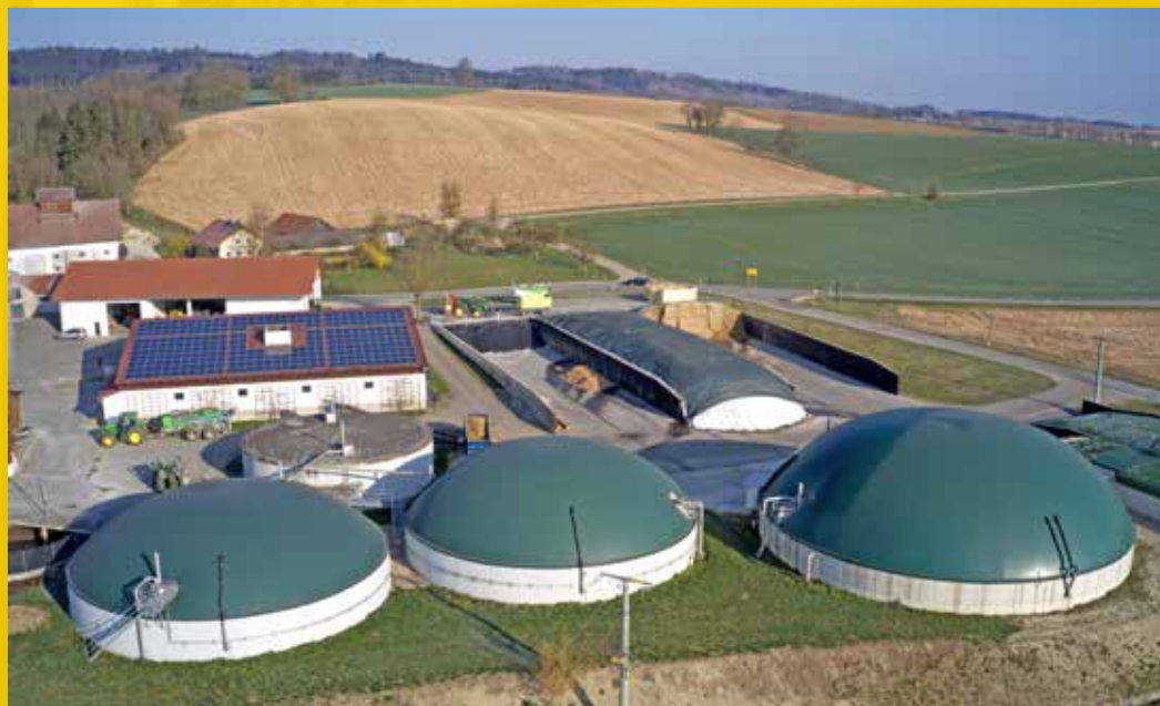
INSTALLATION DE BIOGAZ
