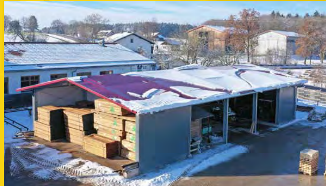
MACHINE HALL WITH CANOPY
