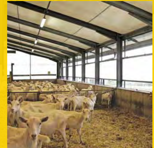
Animal welfare goat house in textile construction method with curtains in shading position
