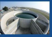
"Aeration tanks are usually constructed at a height of 7 m to 10 m to ensure the most efficient absorption of oxygen"
