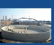
"The floor of settlement tanks is cast at a gradient as specified by the customer"
