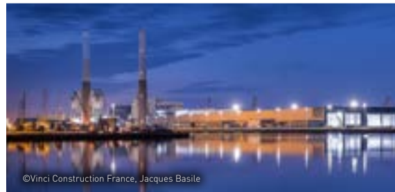
©Vinci Construction France, Jacques Basile
