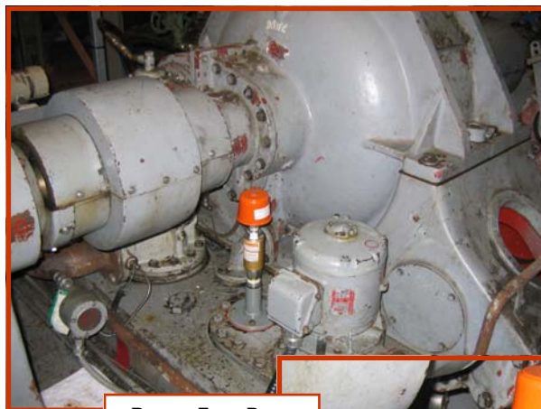
BOILER FEED PUMP FLUID DRIVE COUPLING
