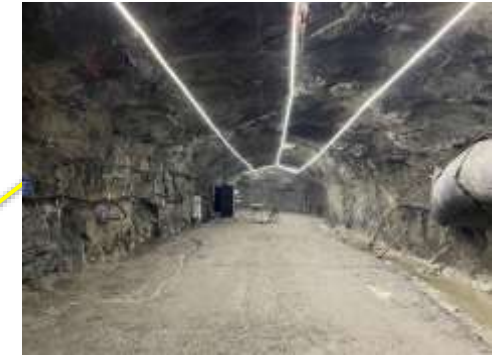
The auxiliary level at -280 m
