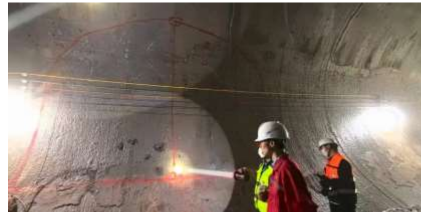
Ramp | Experimental tunnel
