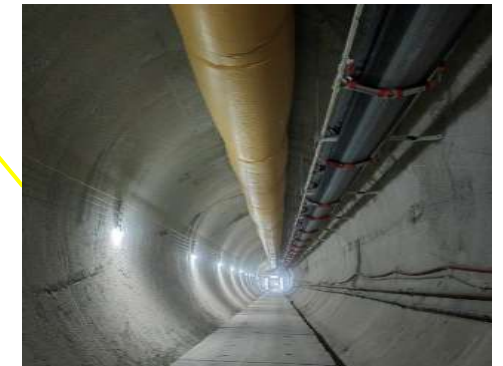
Ramp (4004 m, 15 May 2024)
