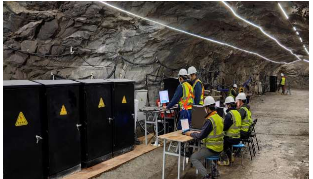
Monitoring at -280m tunnel
