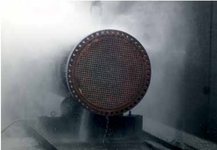
DUST REMOVAL: ± 1 HOUR HIGH-PRESSURE WATER JETTING
