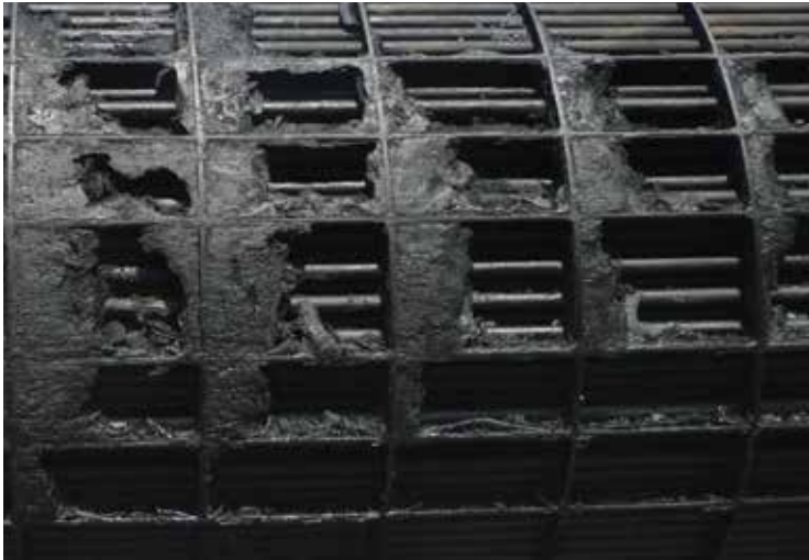
BEFORE THERMAL CLEANING: 100% POLLUTION
