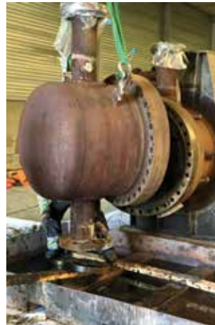
dismantle the heads
