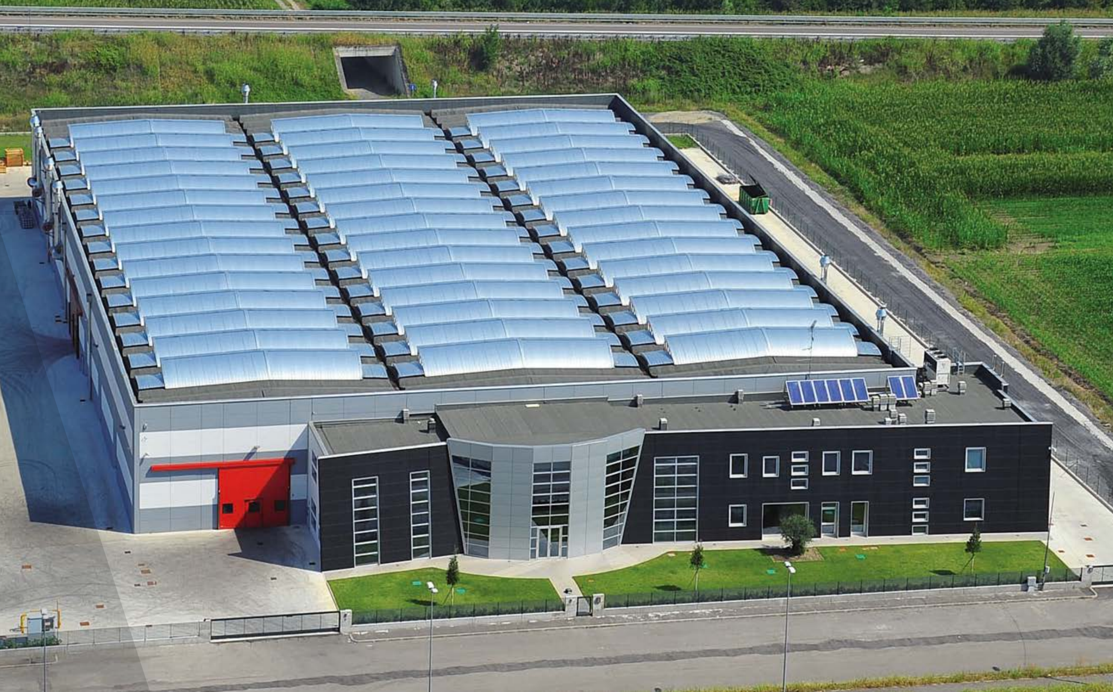
Company Headquarter (Brescello - Italy)
