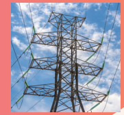
Energy retailers and independent aggregators
