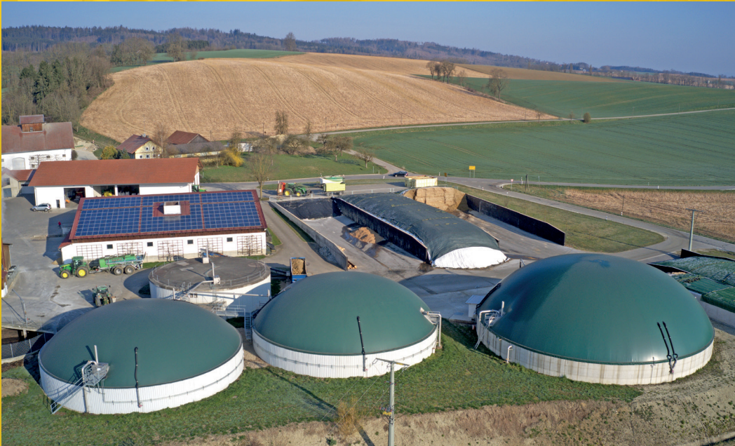
INSTALLATION DE BIOGAZ
