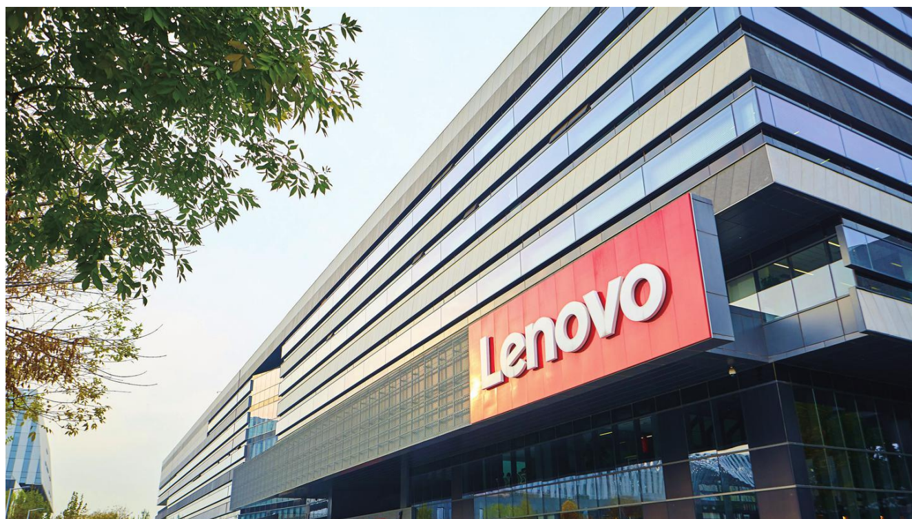
Lenovo's operation center in Beijing, China.
