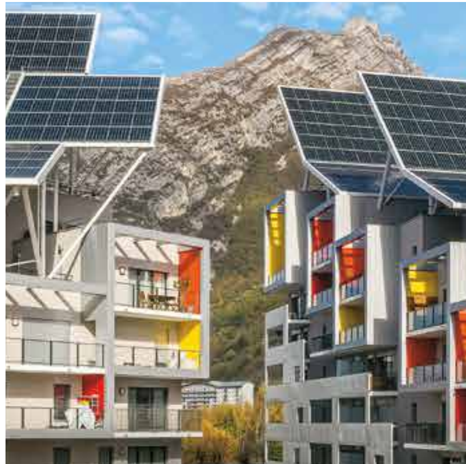
ABC building in Grenoble, France (Autonomous Building for Citizens)
