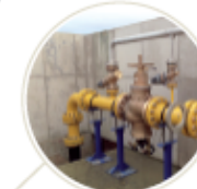
OXYGEN SECTIONING STATION
