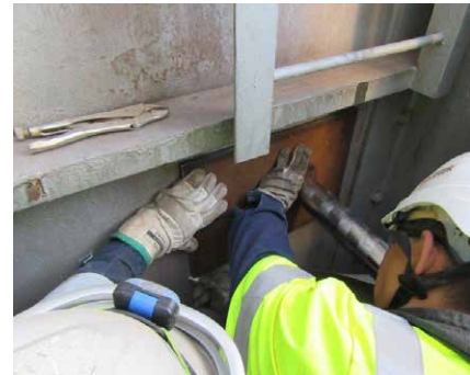
Hot Tube Descaling
