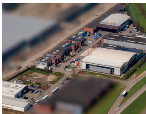
Valk Welding NL
