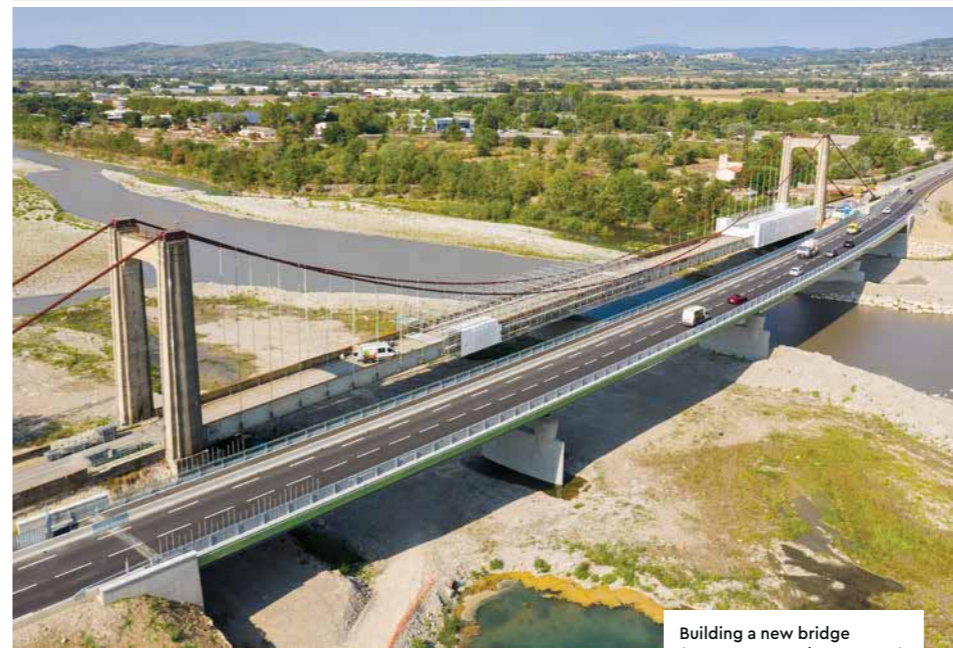
Building a new bridge (Manosque, southern France)
