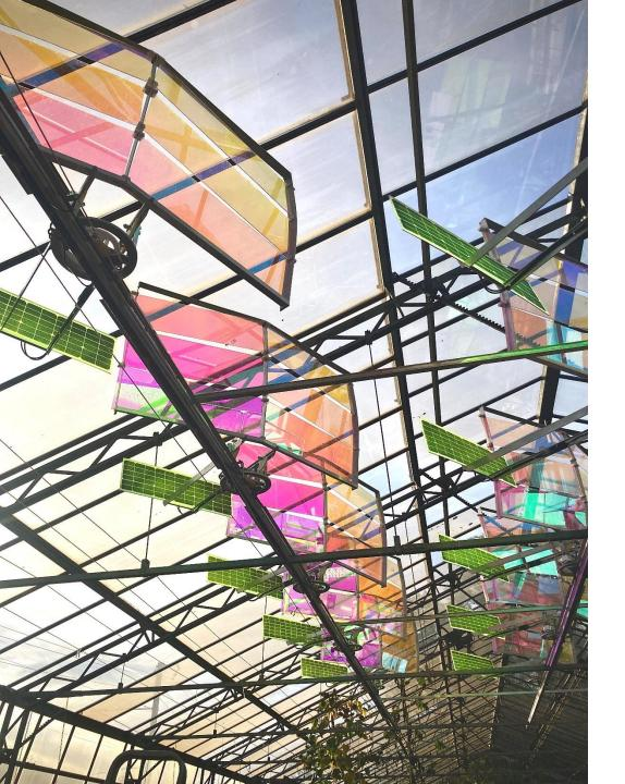
To enable this vision, Voltiris develops the first solar modules for existing greenhouses
