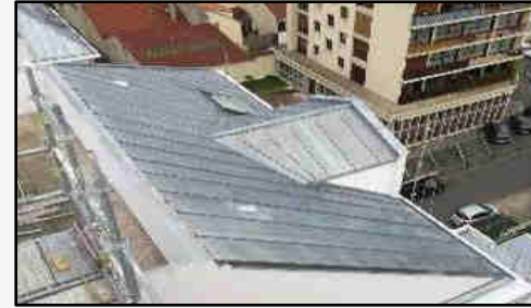
Rue Pierre Curie Alforville (94) - LOGIAL
