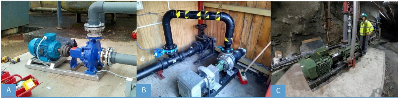
A Turbine at the inlet of a raw water storage tank in a rural Irish water scheme
