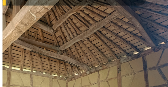
RENFORCEMENT STRUCTURE BOIS
