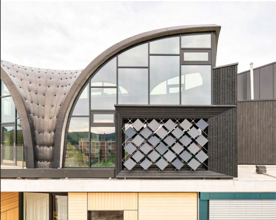
The Adaptive Solar Façade installed at the HiLo unit, NEST in Dübendorf, 2022 © Roman Keller (Zurich)
